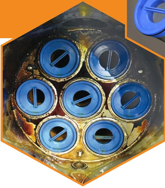
Secondary filter vessel with replacement FTC Torrent 600 pleated cartridges, offering 12 times the surface area of existing bag filters
